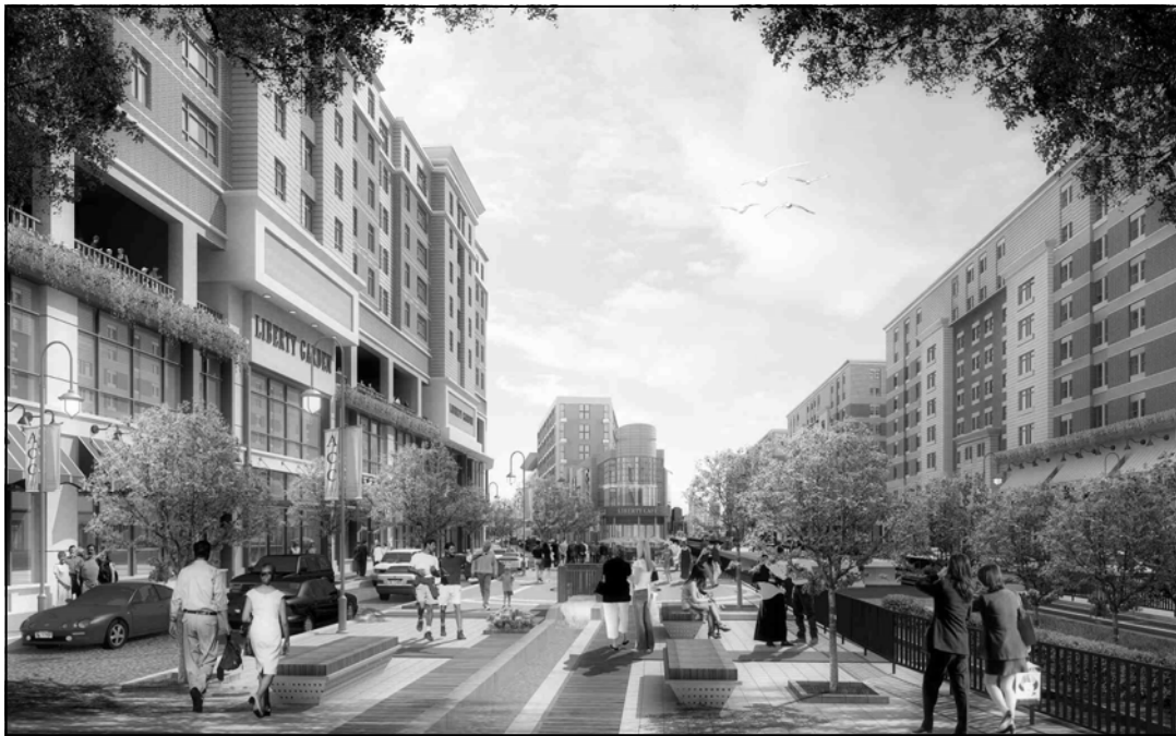
Liberty Harbor is a mixed-use community in downtown Jersey City that will comprise as many as 10,000 homes and 250,000 square feet of retail space. It has a ferry terminal and light rail station.
